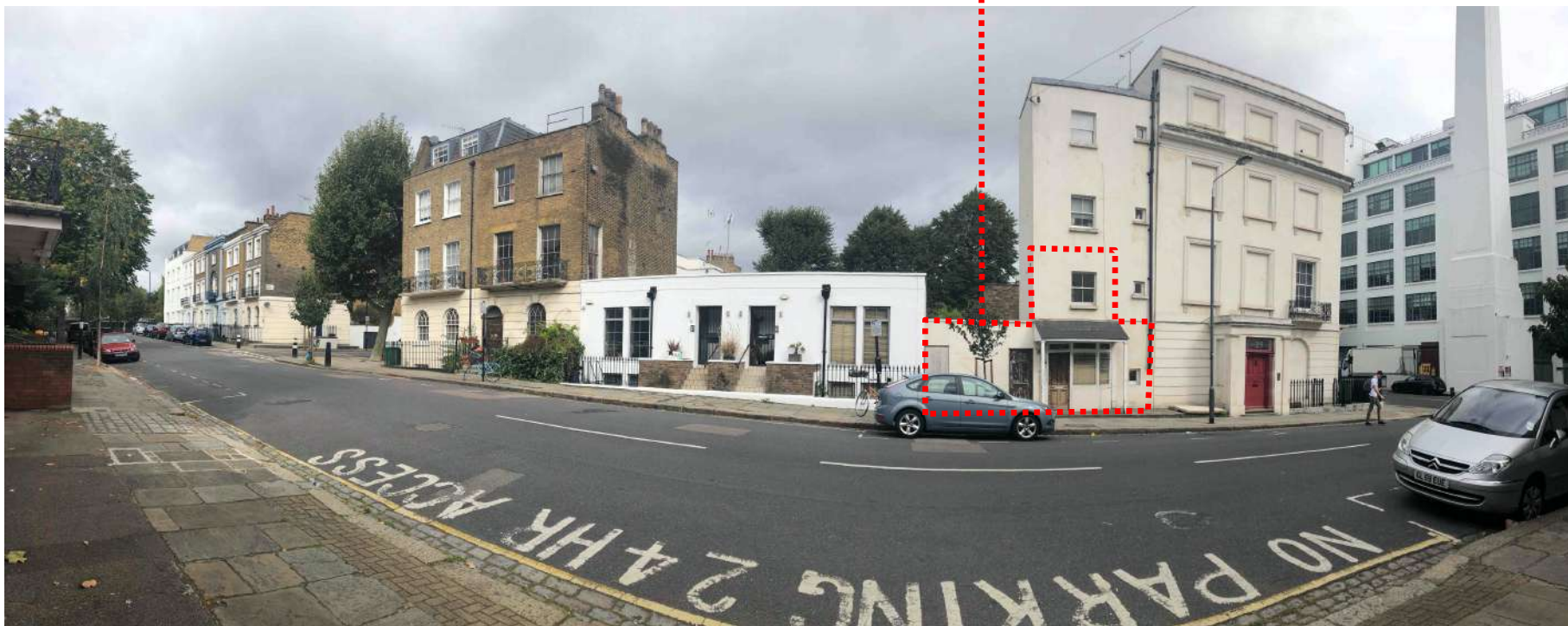
Street scene view to front.
