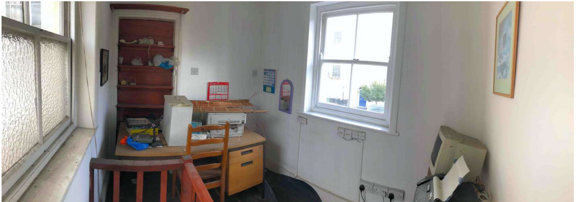
View to currently inaccessible (ladder access only) first floor/mezzanine.
