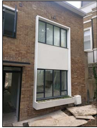
Diagram C Existing projecting architrave at front of 2 Upper Park Road
