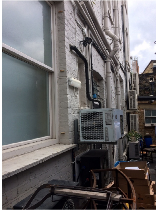
Photo of the Rear Elevation
