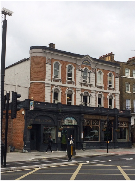
Photo of the Front Elevation
