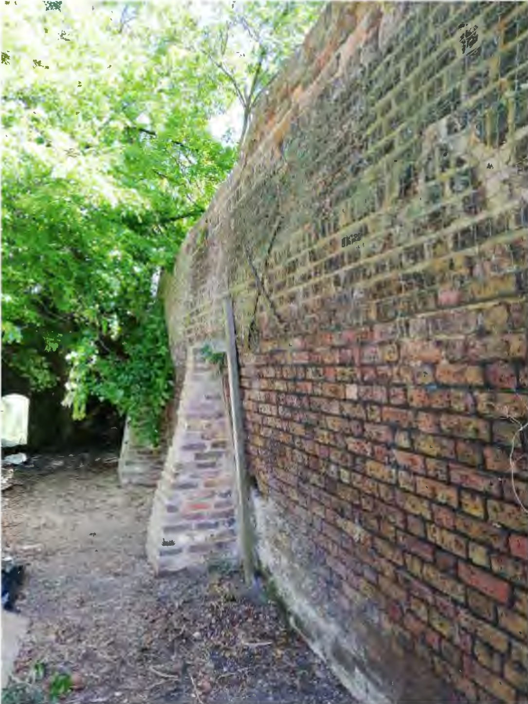
Photo 11, North Section of Wall showing newer piers and bow at the top of the elevation. Also evident is the anchor plate situated in front of the nearest pier.
