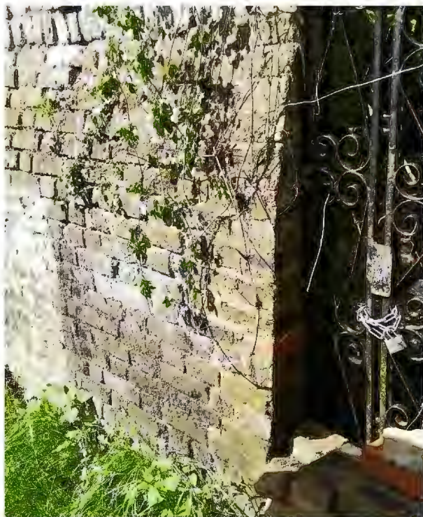
Photo 5, new/old brickwork at opening reveal
