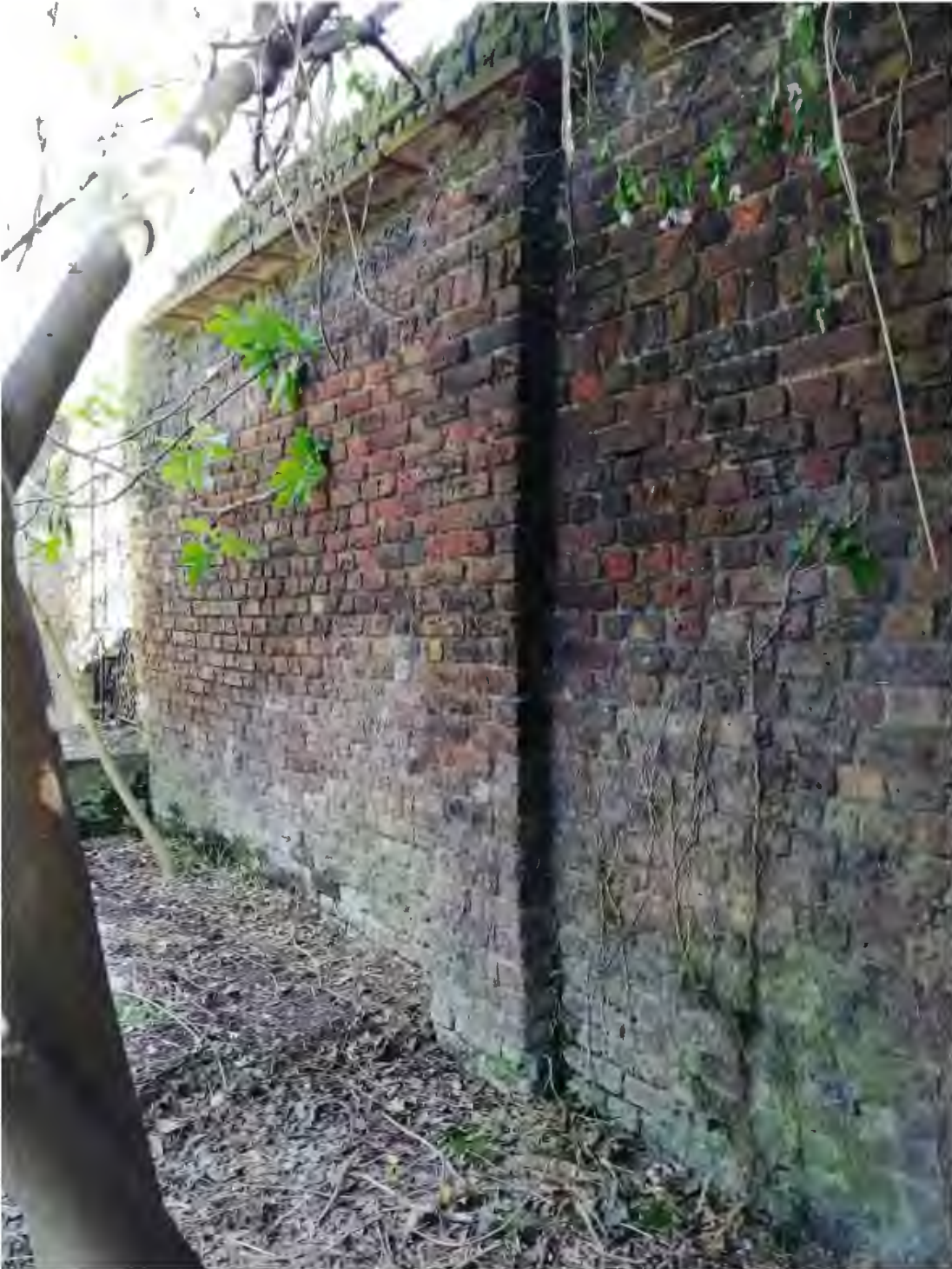
Photo 13, Elevation 4, RHS of opening on 22 Frognal Way side
