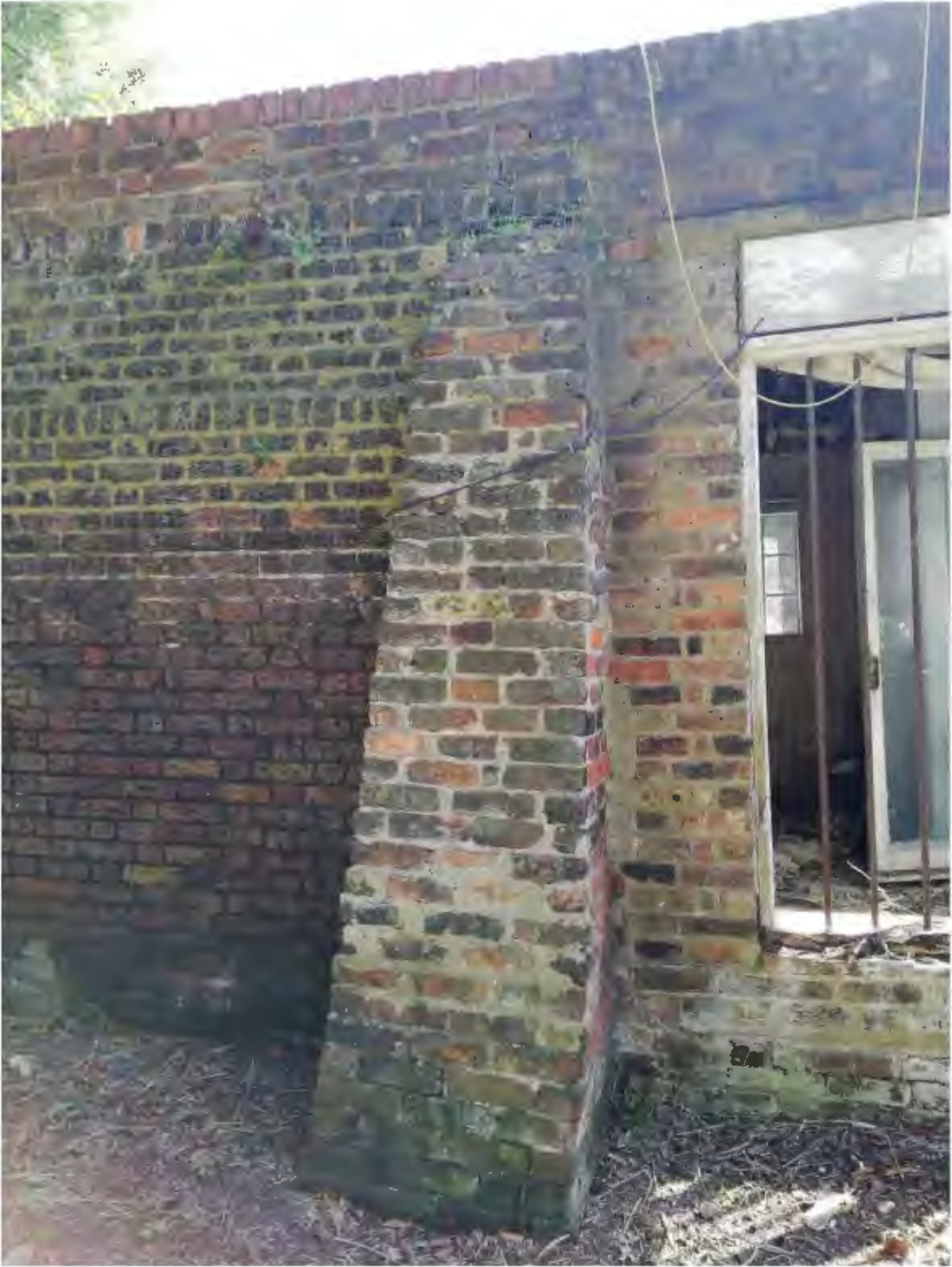
Photo 10, Right-hand side masonry pier to Outbuilding
