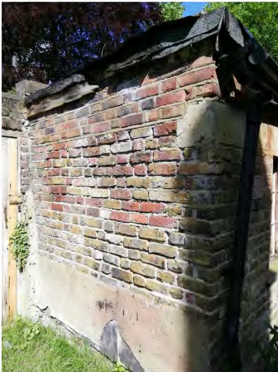
Photo 8, View of Outbuilding Masonry
