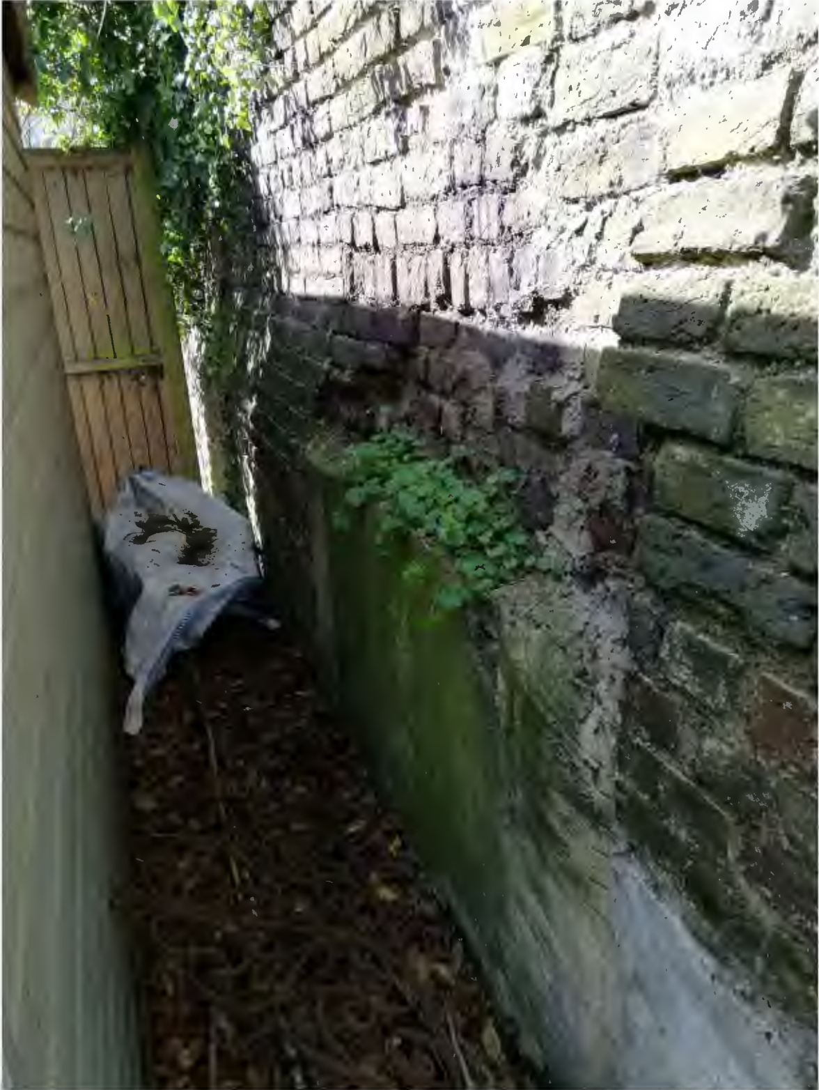
Photo 2, Southern section of wall behind existing shed
