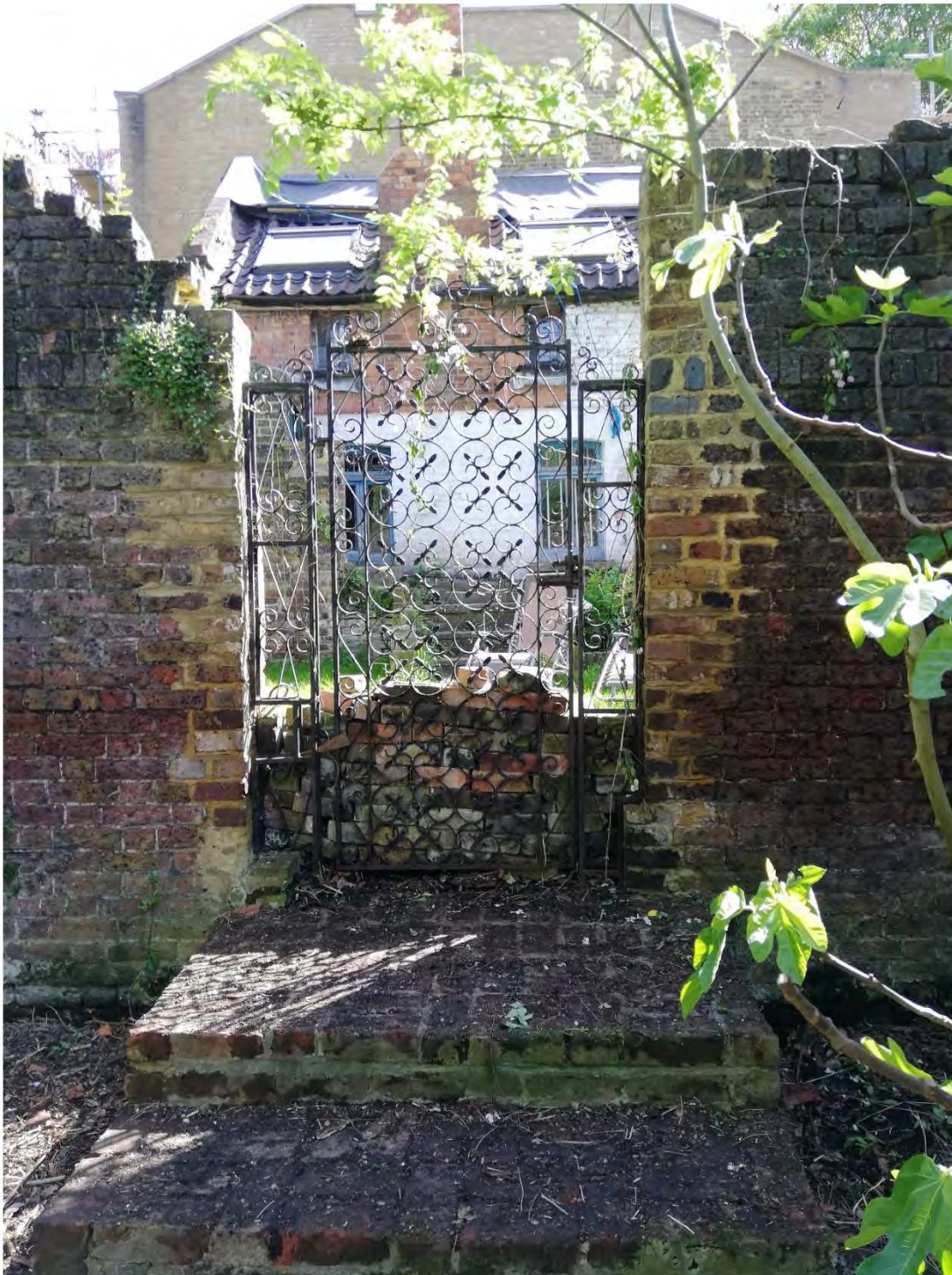
Photo 15, Opening 1 with new brickwork evident
