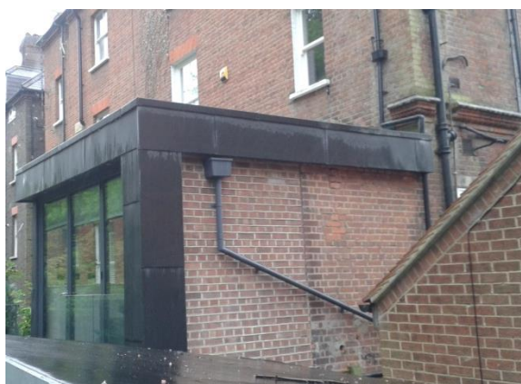
Rear conservatory ~2010 showing movement joint - not in new add-on
