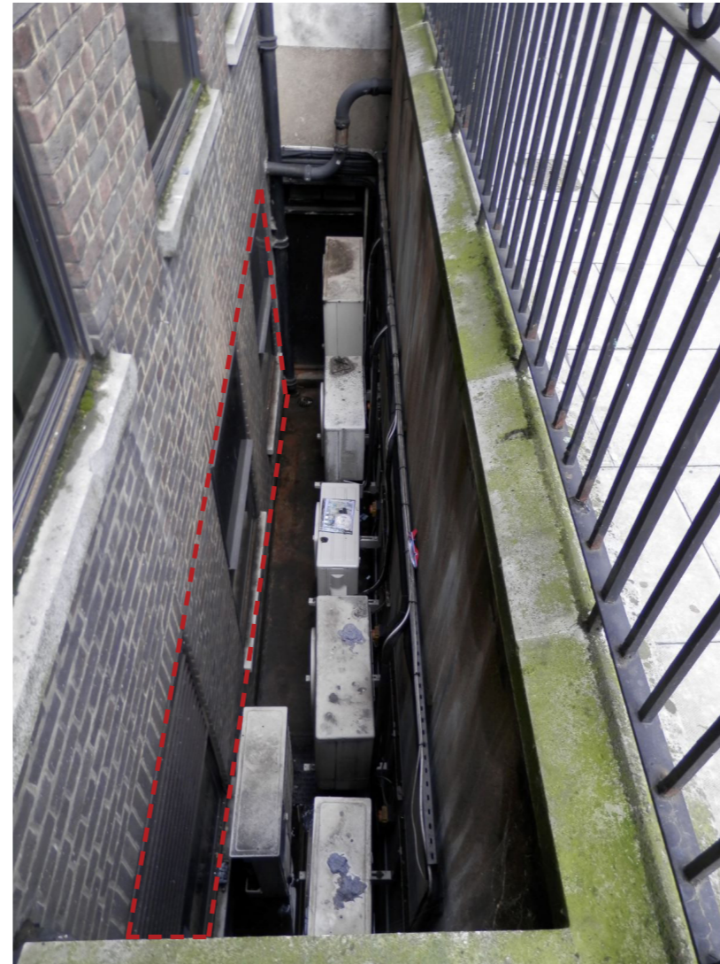
--- Location B - Basement unit can utilise Lightwell for filtered extraction Details of ventilation model and filtration to be submitted by future tenant under planning condition
