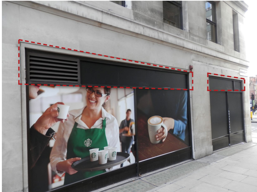
--- Location A - Ground floor unit can utilise high Level band in shopfront for filtered extraction along Warwick Court Details of ventilation model and filtration to be submitted by future tenant under planning condition
