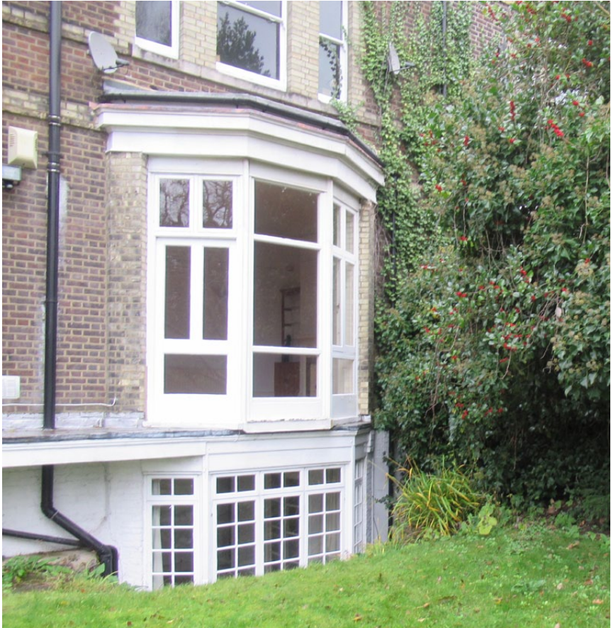
p) View of existing re-built main rear bay, redundant platform, un-orderly soil pipes and satellite dishes
