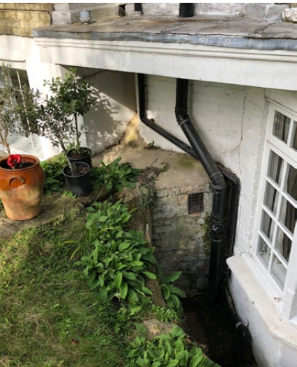
r) vented void infill to rear areaway to be removed
