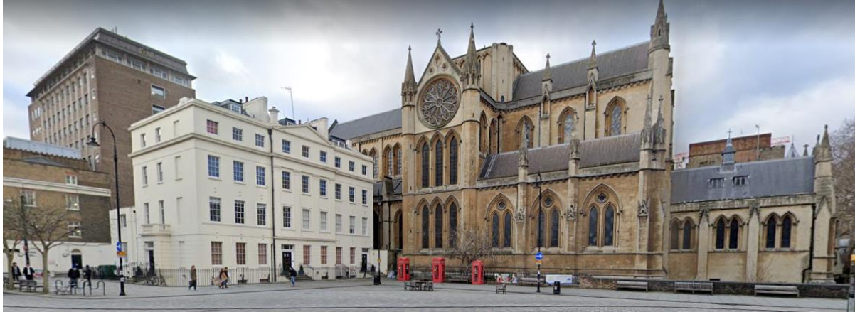
5. View from Torrington Square with the 4 storey building concealing the MPBE Building behind
