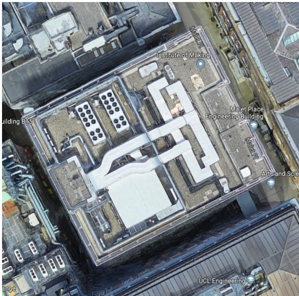
1. Rooftop view of existing MPBE Building
