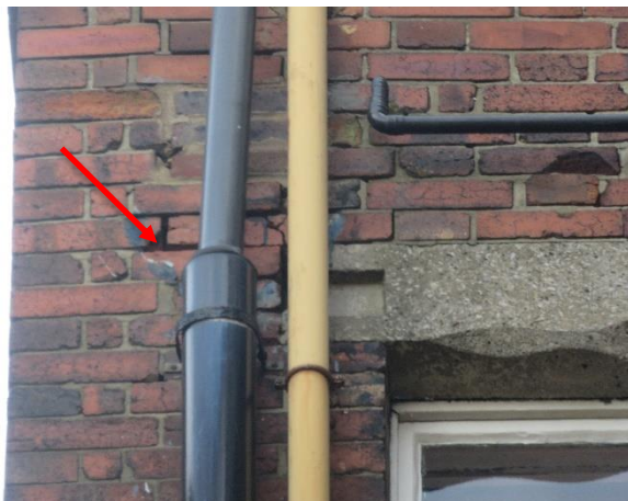
Plate 4.5: Gaps in brickwork
