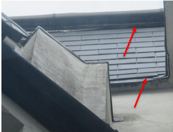
Plate 4.3: Gaps under Hanging Tiles and Lifted Lead Flashing, Viewed from Internal Courtyard
