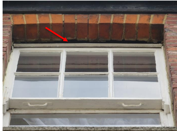
Plate 4.4: Gap between Window Frame and Brick Lintel
