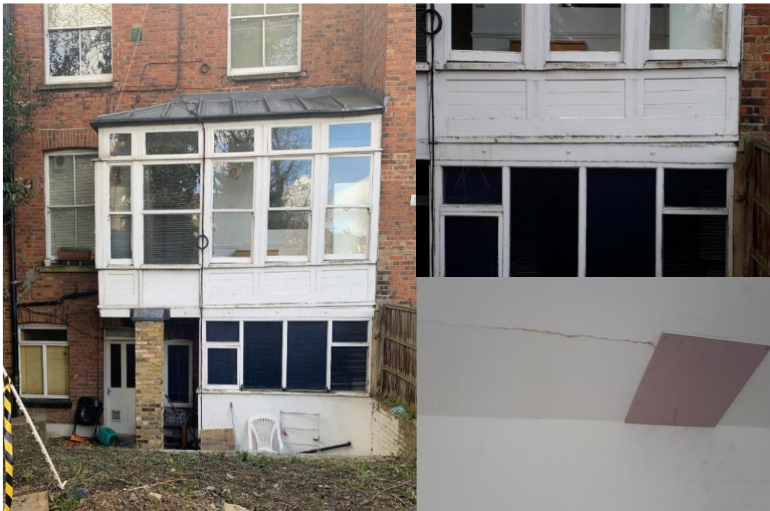
EXISTING REAR EXTENSION
