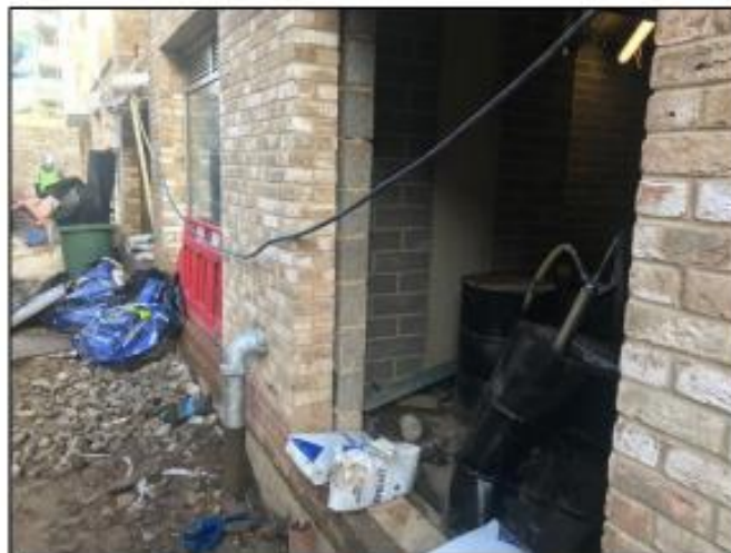
Figure 5 - Dry Riser Pipework entering Building C
