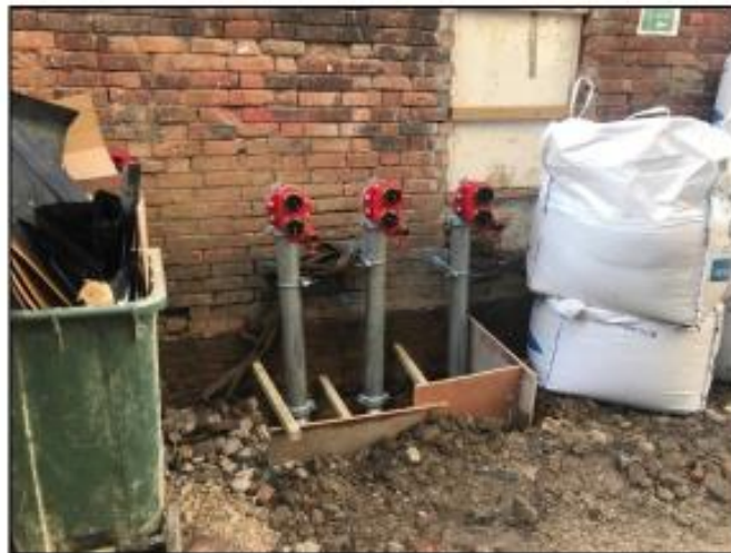
Figure 4 - Dry Riser Inlet Connections and Pipework
