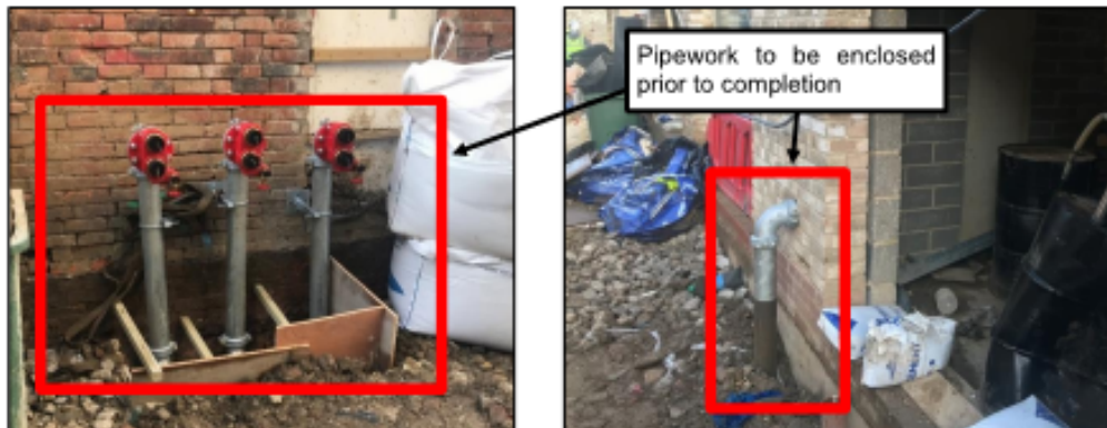
Figure 6: Enclosure to pipework
