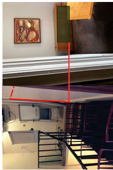
High level CHW and LTHW pipework path along the wall in the Provost Dining Room. Indicative FCU shown in green, locations are not exact
