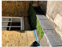
Indicative route of condensate pipework in blue from Provost's Dining Room and Whistler Room
