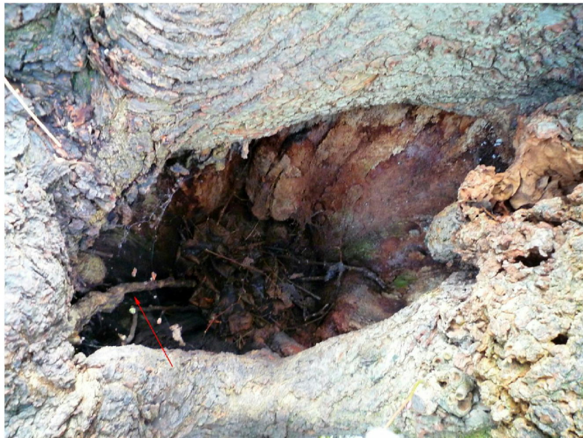
4) Closer view showing decaying side walls and accumulated leaf litter / compost. Arrow shows an adventitious root growing into this material.
