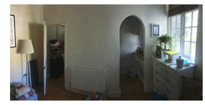
Non structural kitchen partition (added during conversion to a flat), to be removed . Note that it obscures the window. The door which is also contemporary with the added partition is also to be removed ( along with the radiator) Like the rest of the flat, there are no surviving original architectrual mouldings. The WC is proposed to be relocated in the bathroom and the space used to improve the kitchen
