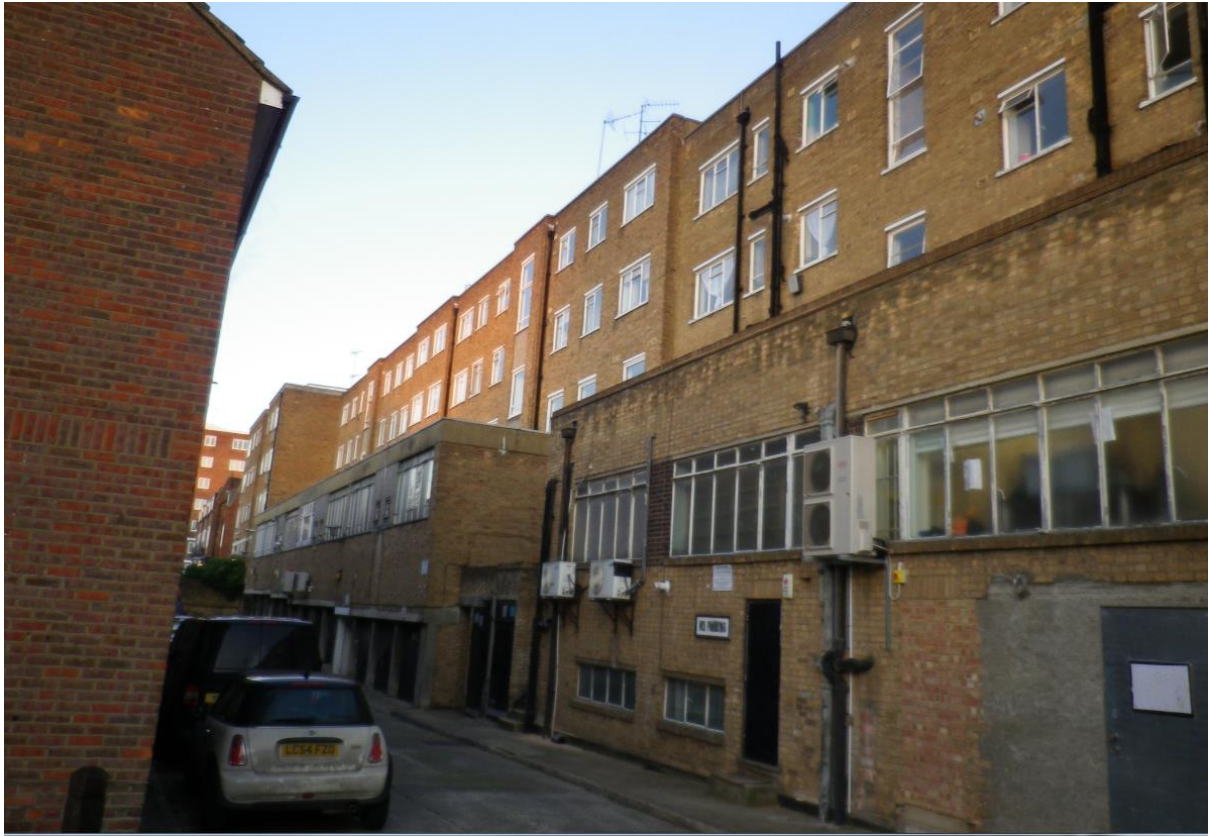
Photo 3: Rear service area on Fairfax Place
