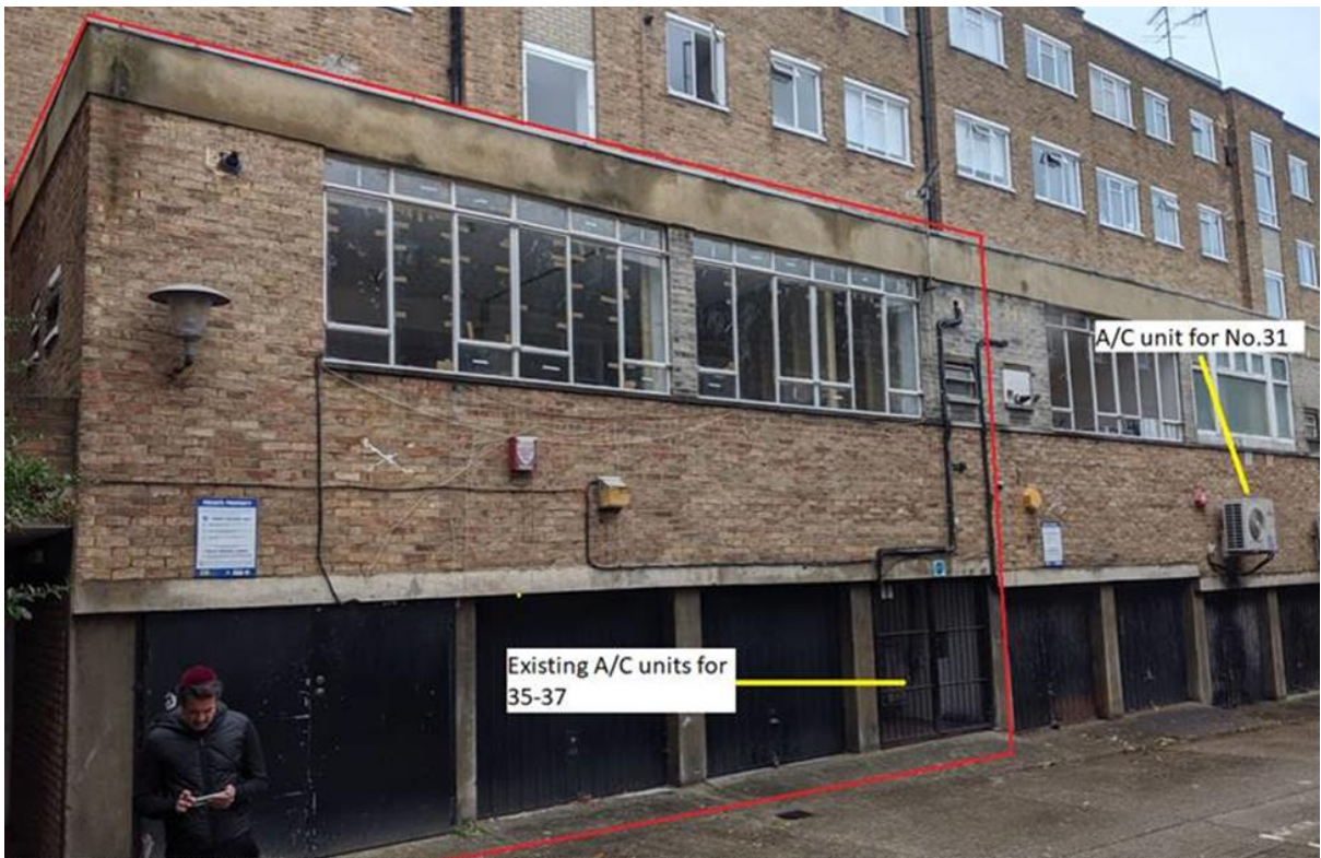
Photo 4: Rear elevation fronting onto Fairfax Place
