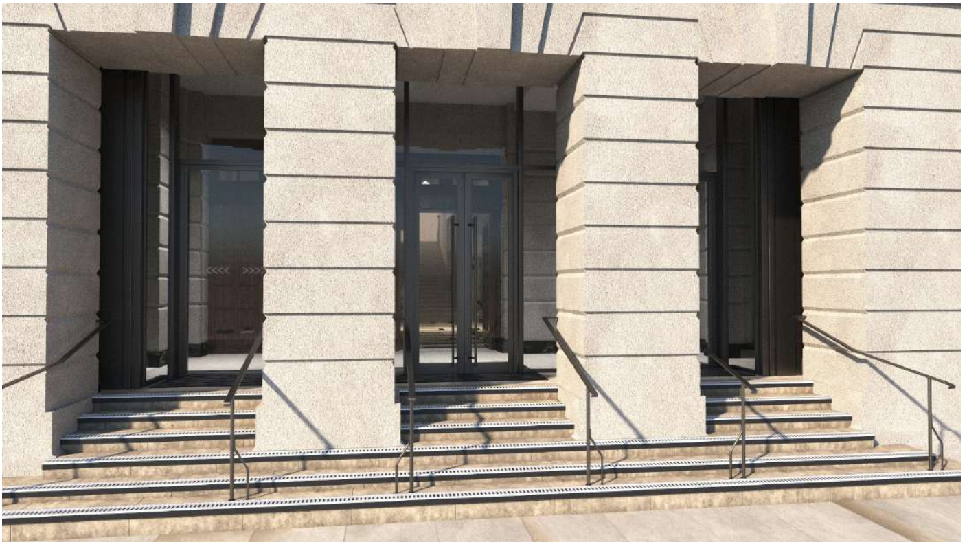
Proposed Judd Street Entrance - visual showing rebuilt stairs with contrast nosing and new glazed entrance lobby
