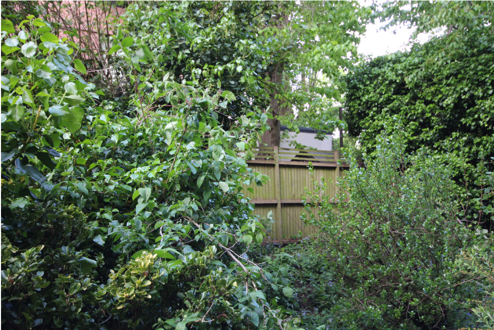
View of boundary fence from public entrance pathway to 42 - 51 Clevedon Mansions
