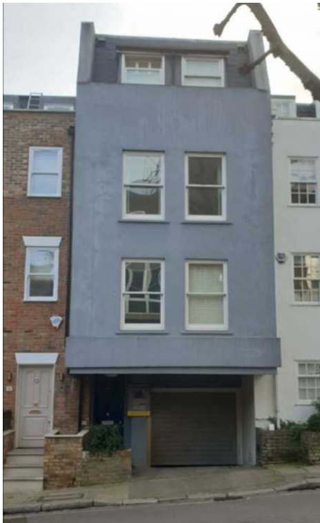
1 (above): Existing front elevation
