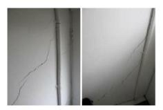
To the first floor, cracking is present to the sitting room front wall below the window and is also present to the stairway to the second floor, with cracking to the wall / ceiling junction and adjacent the window cill of the front wall.
