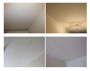
Further cracking is present to the ceiling of the front central room, extending longitudinally back from above the window opening, although this is less pronounced.
