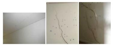
Cracking is also present within the front left-hand side room, largely manifesting at the wall / ceiling junctions, although cracking is also present to the rear wall at the rear left-hand side corner.
