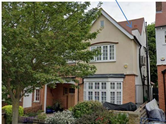
Opening up works and the erection of the scaffold externally have allowed closer inspection of the existing building to review repair needs. Inspection revealed the extent of cracking to the front chimney was beyond minor brick stitching and piecing in repair. It has been necessary to take the chimney down temporarily for safety reasons.
