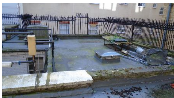
12. Failed roof covering to first floor
