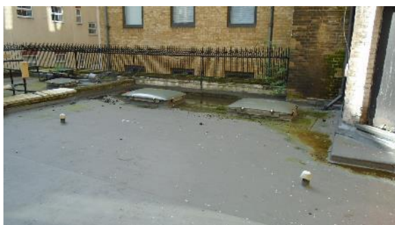
11. Failed roof covering to first floor
