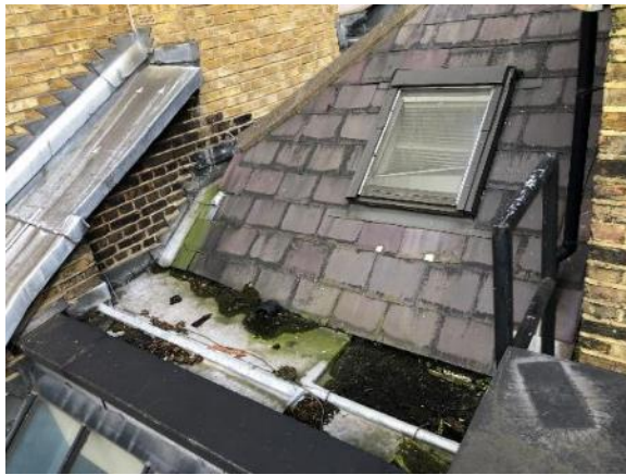
7. Lead box gutter
