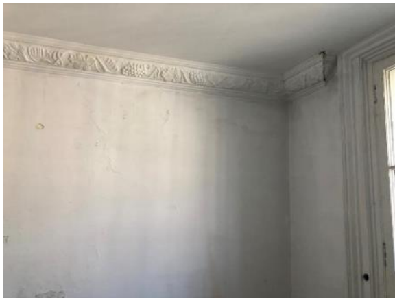
13. Visible water ingress to internal accommodation at third floor
