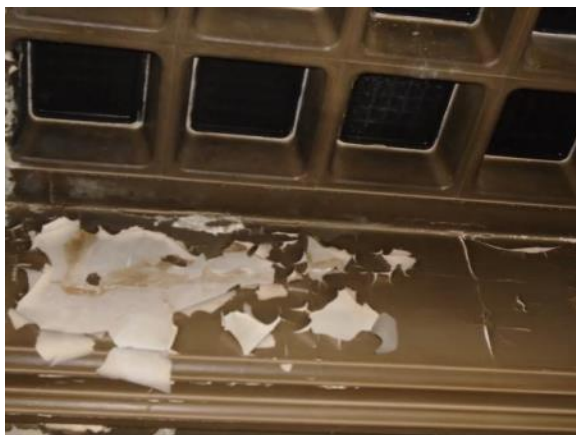
15. Visible water ingress to internal accommodation at ground floor
