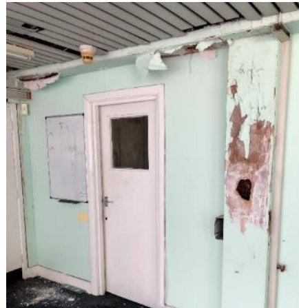
14. Visible water ingress to internal accommodation at third floor
