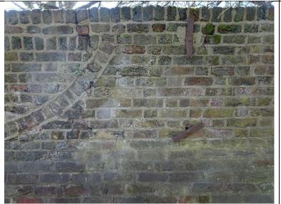
Wall has been extended upwards above the original curved profile. Irregular bond pattern.
