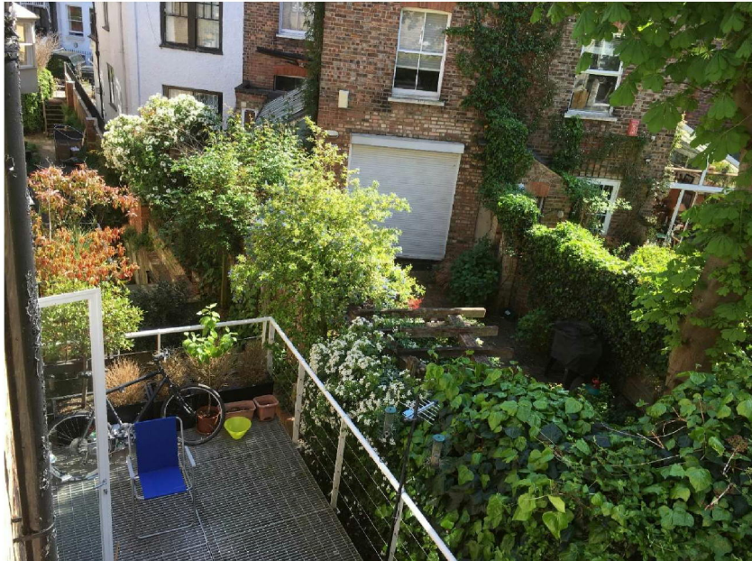
PHOTOGRAPH 01: View showing close abutting relationship of Rear 31 Willoughby Road with Rear Access and Amenity spaces of Registered Heritage Assets Grade II Listed Willow Cottages and lower rear boundary retaining wall looking east
