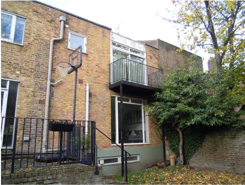
3. rear showing basement room window
