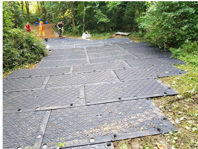
Inset 3: Interlinked ground protection boards placed on top woodchip
