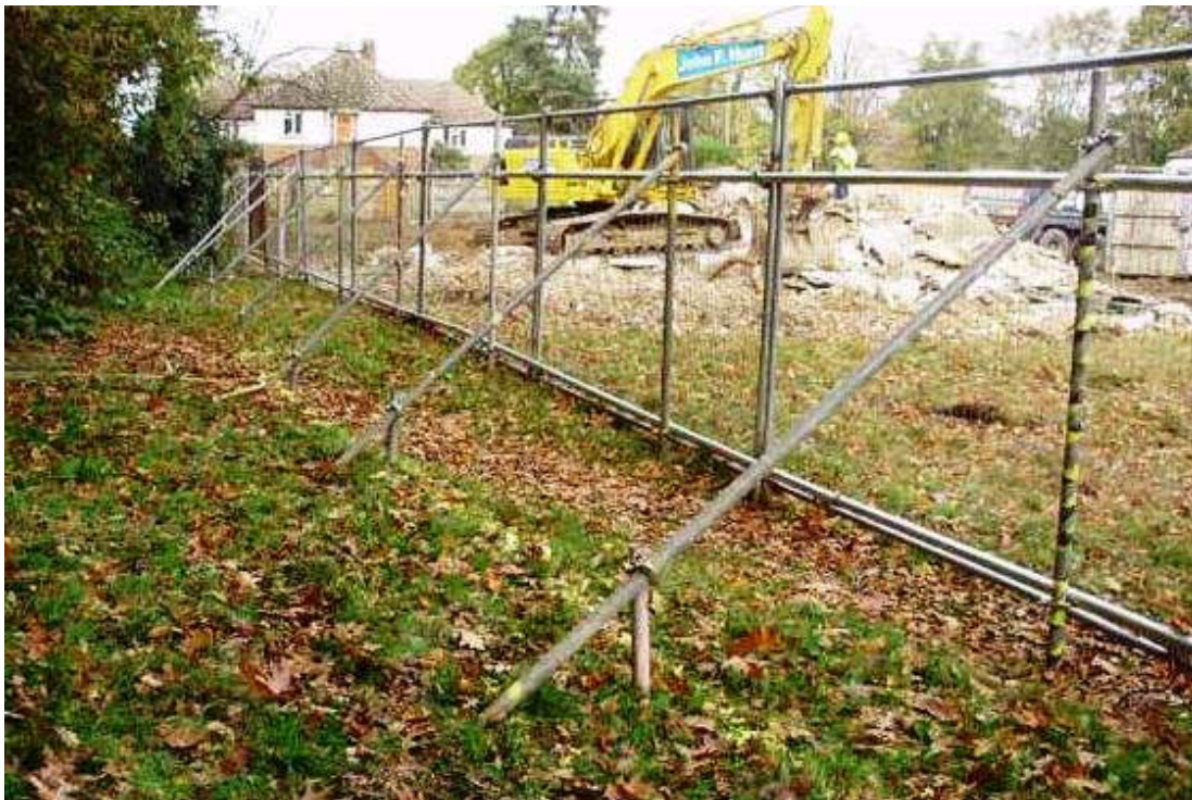
Figure 2: Photo of Fencing to BS 5837:2012
