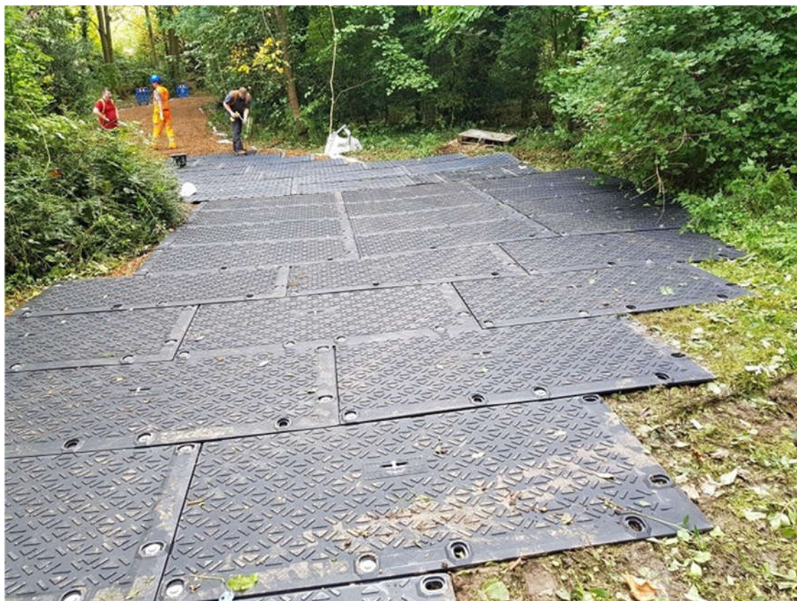
Figure 5: Inter-linked ground protection boards placed on top woodchip
