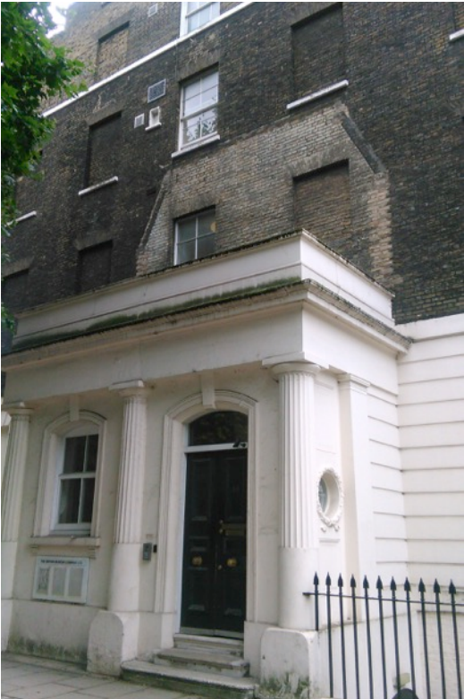
Top: Front Basement yard. Brickwork walls to be cleaned, repaired and repainted. Left: Side Basement yard. Existing stone staircase and York stone paving to be cleaned and repaired. Essential maintenance works to be carried out to unblock drainage gullies. Right: Entrance portico to be cleared of organic growth, repaired and redecorated. Brickwork to main elevations to be toned down to match existing patina..
