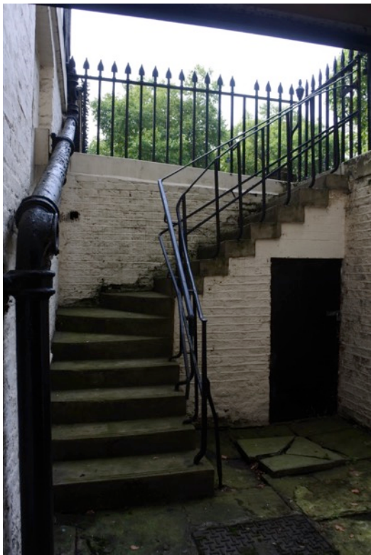
Top: Front Basement yard. Brickwork walls to be cleaned, repaired and repainted. Left: Side Basement yard. Existing stone staircase and York stone paving to be cleaned and repaired. Essential maintenance works to be carried out to unblock drainage gullies. Right: Entrance portico to be cleared of organic growth, repaired and redecorated. Brickwork to main elevations to be toned down to match existing patina..
