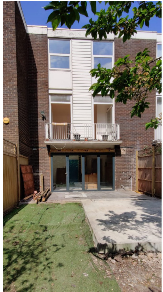
Fig 2. 10 Hornby Close, Existing Rear Elevation
