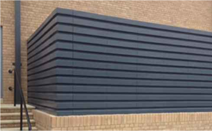
Example 2: Acoustic louvred wall
