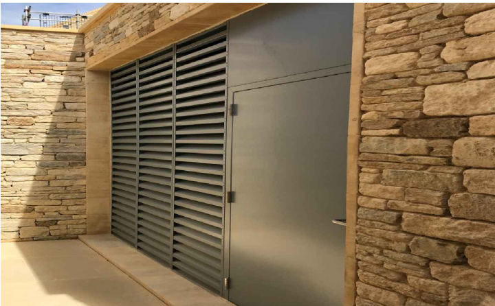
Example 1: Acoustic enclosure with door
