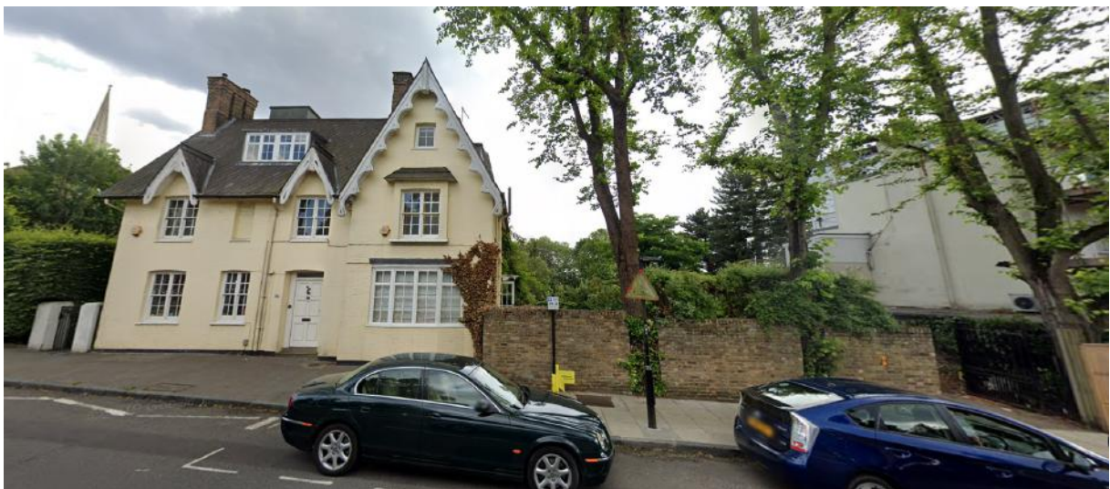
2) Front elevation showing existing access door and boundary wall
