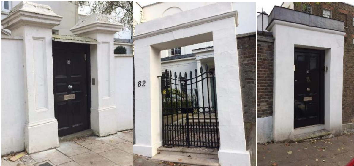
4) Comparable 'breaks' in boundary walls at nos. 81, 82 and 83 Highgate West Hill
