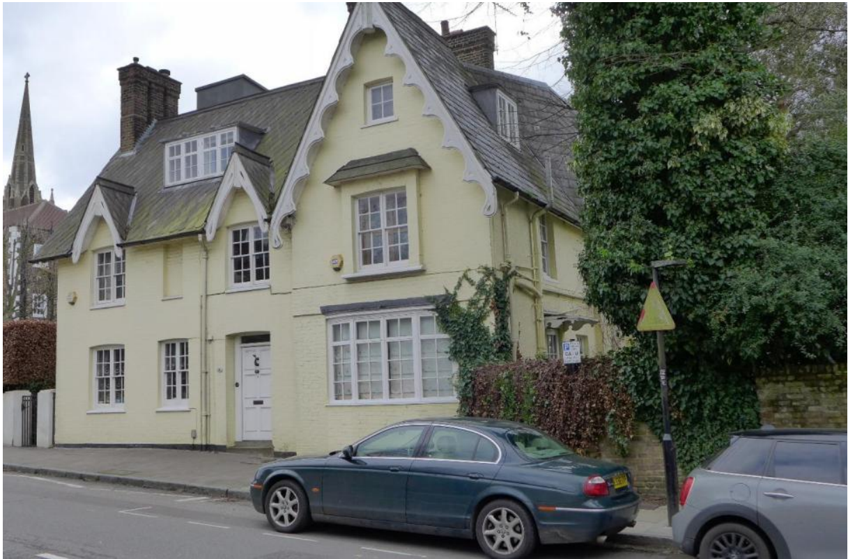
1) Front elevation showing existing access door and boundary wall
