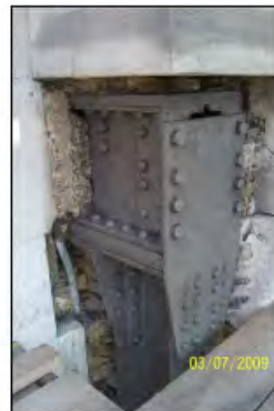
STEEL COLUMN CLEANED AFTER SHOT BLASTING PRIOR TO PAINTING
