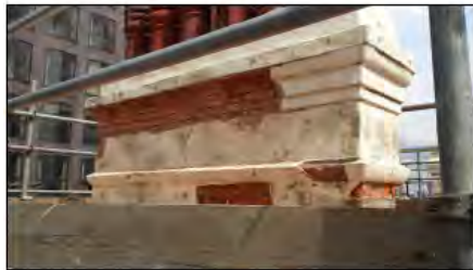
TYPICAL CHIMNEY STACK REPAIR USING HELI BARS
