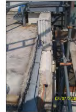
STEEL PARAPET BEAM AFTER CLEANING + PAINTING
