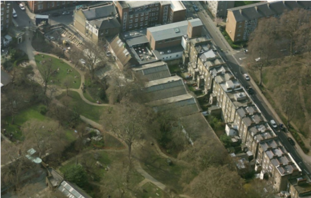
2. Site looking west ^
