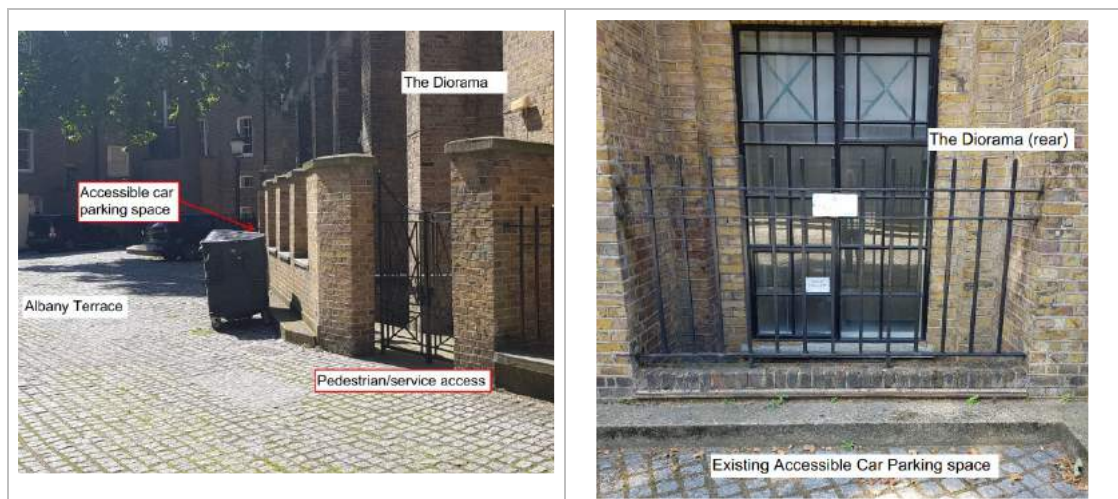
Figure 3.4 – Existing Rear Pedestrian/Service Access and Accessible Car Parking Bay
