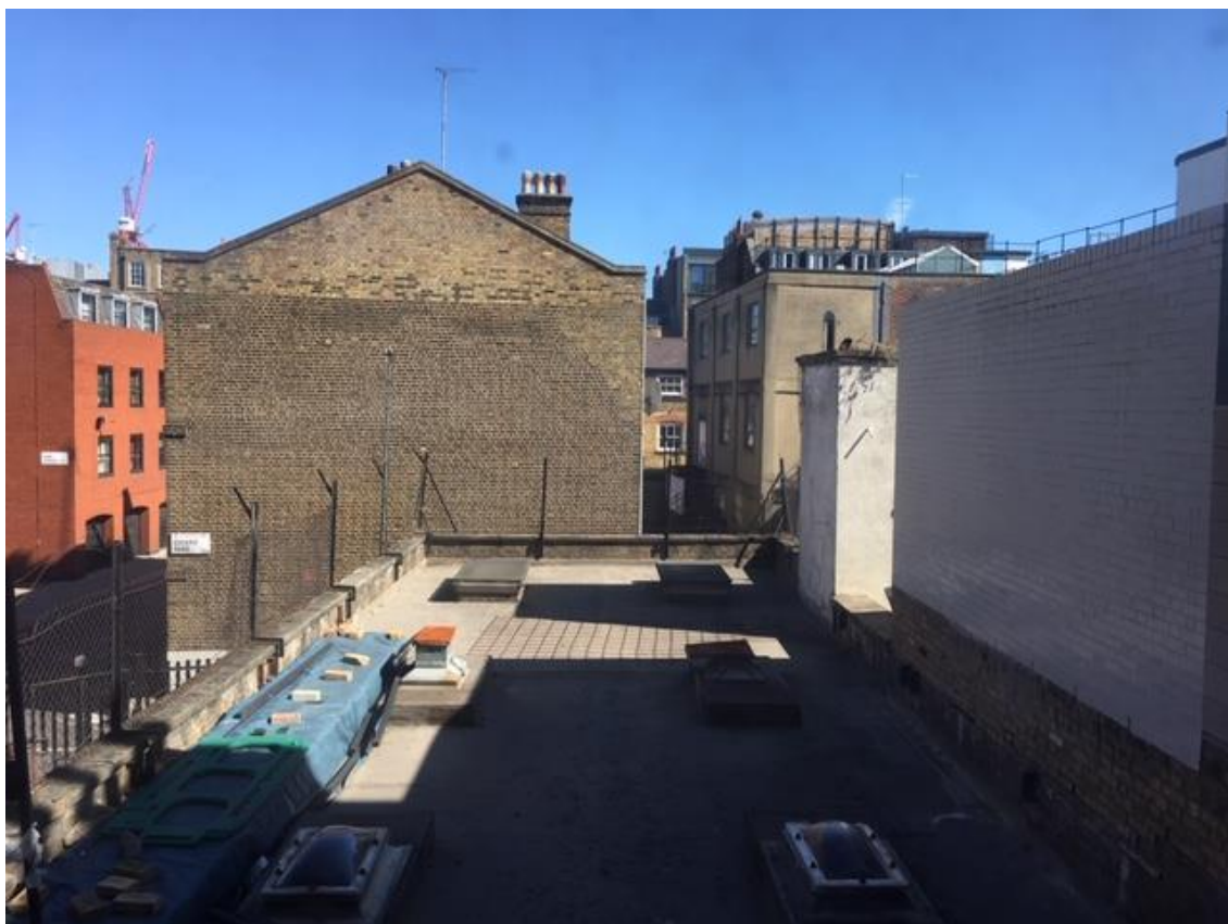
4. Roof top above no.15 ground floor extension
