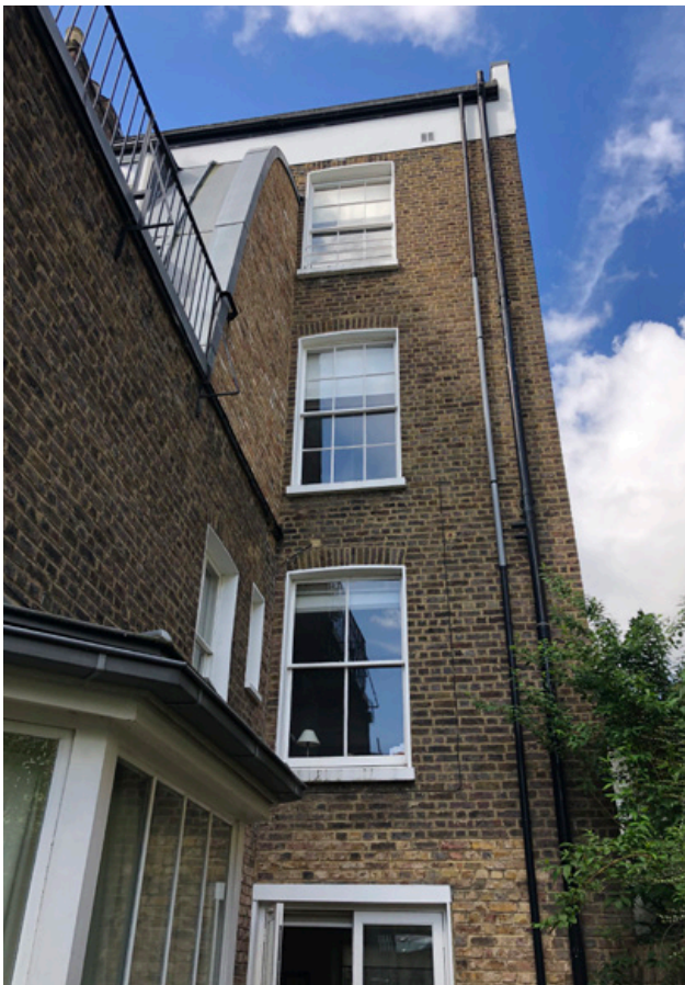
(L) Zinc clad extension showing curved roof
