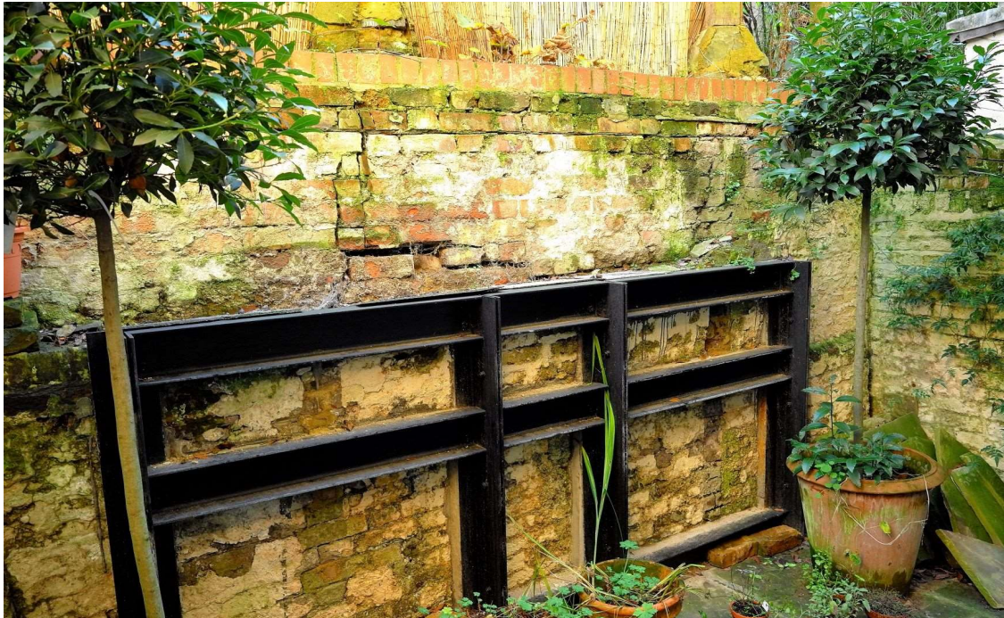
PHOTOGRAPH 03: View showing temporary steel support to damaged lower listed retaining wall as caused by additional loading from raised garden of 31 Willoughby Road.
