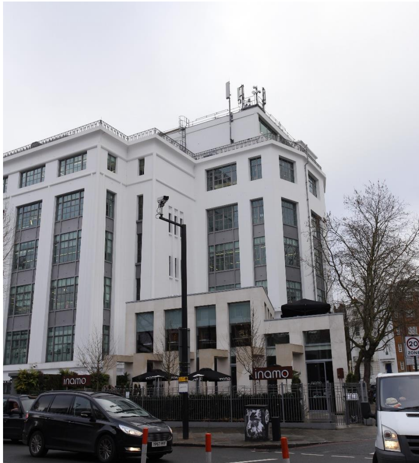
Photograph of the northern end of Greater London House
