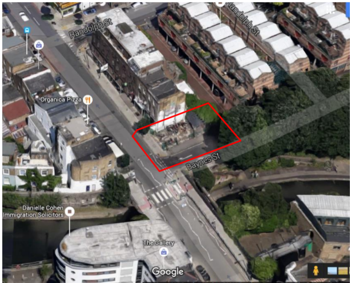
Photo 1: Aerial view of the site
