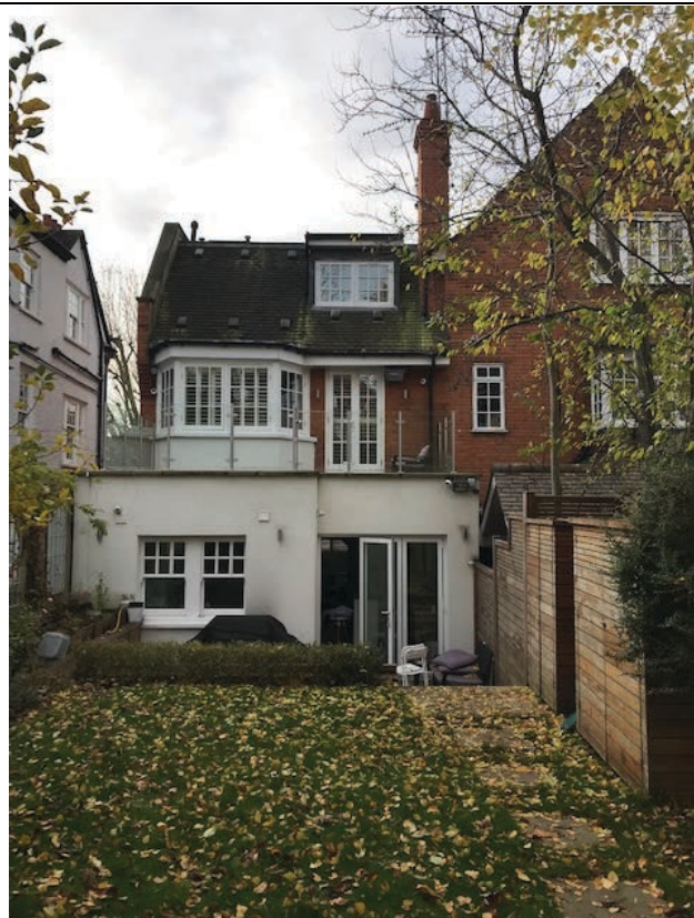
Rear views of existing extension of 20A Ferncroft Ave
