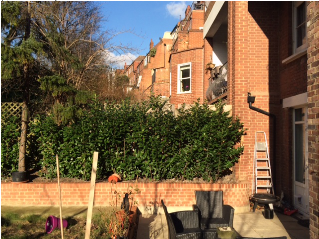
(5) Rear building line of nos. 7&9
