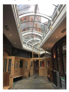
Fig 1 The existing barrel vaulted infill structure looking south through the ground floor reception area.
