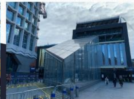
Tottenham Court Road Station
