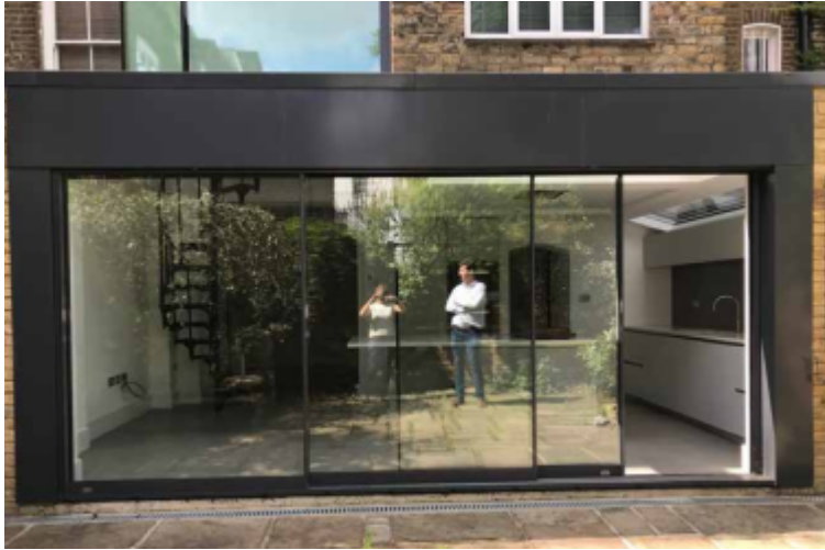
Photograph 4 – Existing lower ground floor
