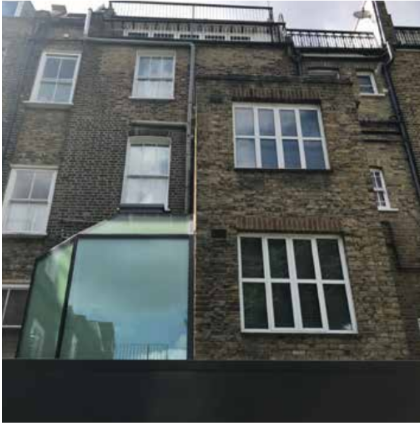
Photograph 2 – existing rear façade
