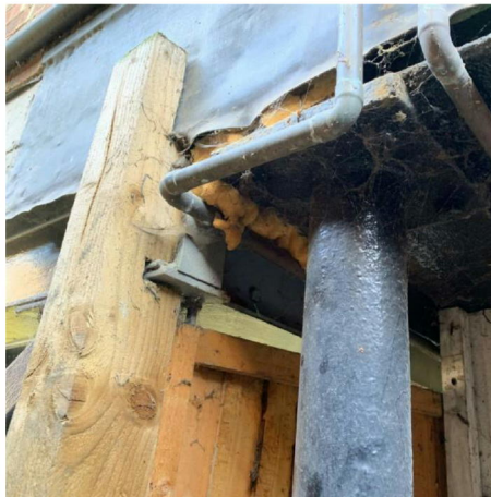
Supporting columns to original projection
