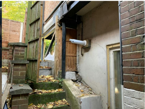
Supporting column to original projection and diagonal crack on lower ground flat wall
