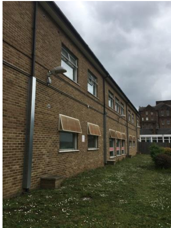
Photo 10. Eastern elevation of Ash House (B3).
