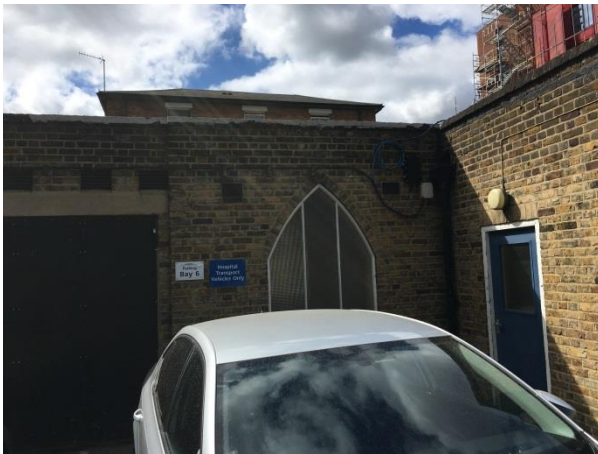
Photo 13. Flat roof on the Mortuary building (B5).
