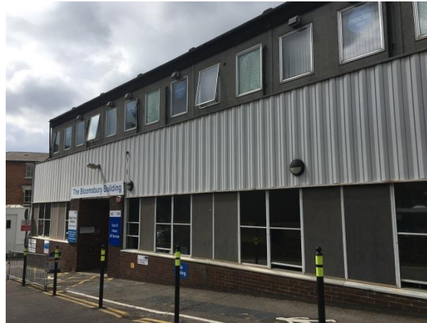
Photo 11. Southern elevation of the Bloomsbury Building (B4).
