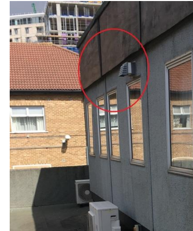
Photo 12. Gaps under the soffit at the northern elevation of the Bloomsbury Building (B4).
