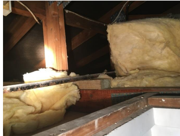
Photo 5. Roof void of Jules Thorn (B1).
