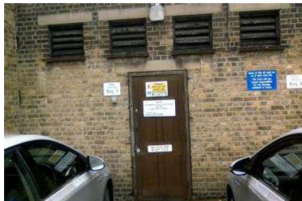
Photo 14. Switch room in the Mortuary building (B5).
