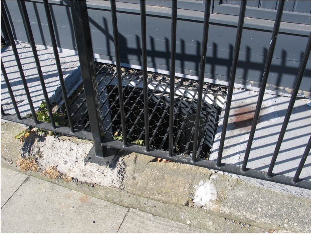
Basement flat: grille above window to bedroom
