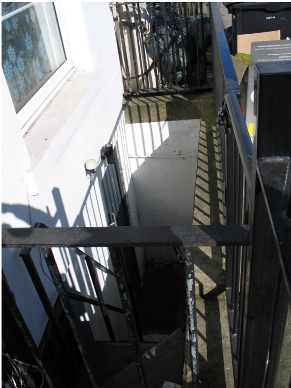
Basement flat: steps to front entrance door
