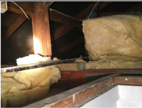
Photo 5. Roof void of Jules Thorn (B1).
