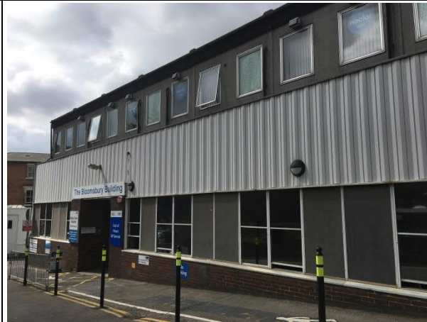
Photo 11. Southern elevation of the Bloomsbury Building (B4).
