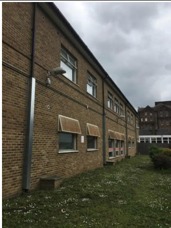
Photo 10. Eastern elevation of Ash House (B3).
