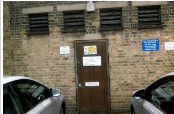
Photo 14. Switch room in the Mortuary building (B5).
