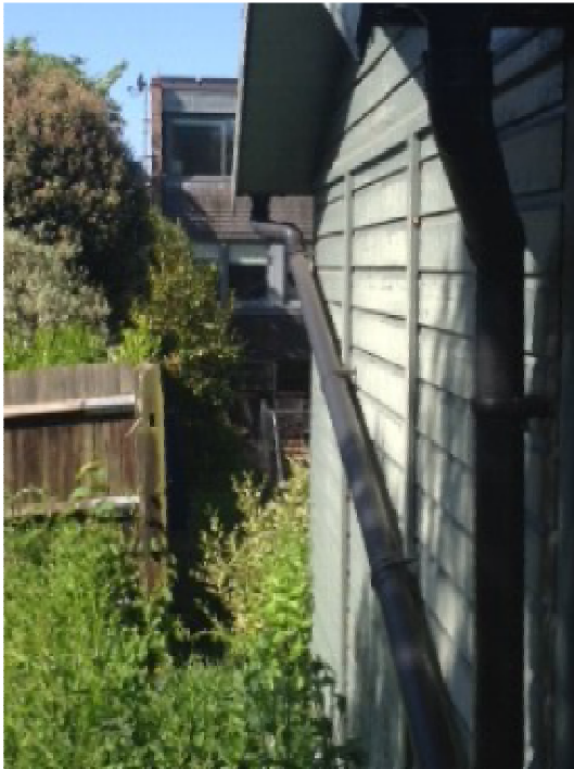
Photo 4 – junction of ‘L-shaped’ boundary fence (facing house at no.4a)
