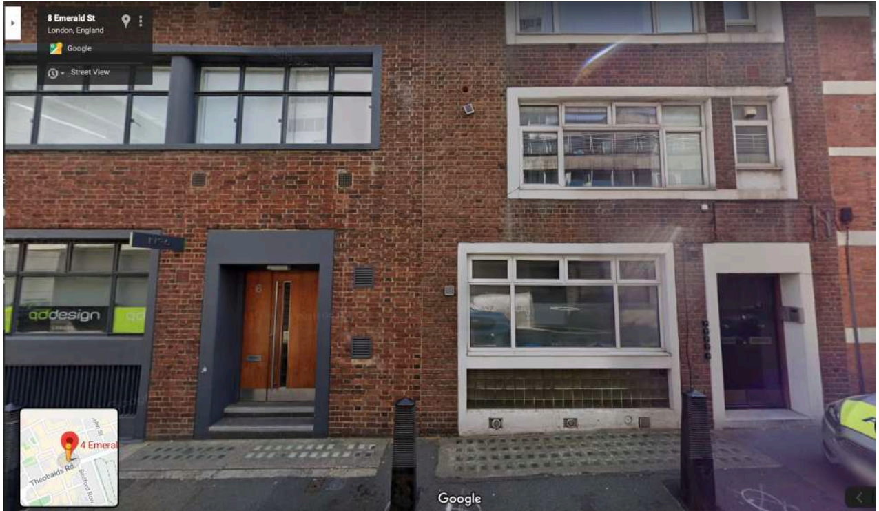
Front view of entrance doors at No.4 Emerald Street with adjacent No.6-8.
