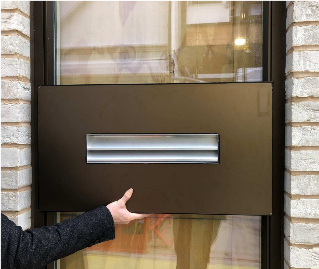
Mock-up of Spandrel Vent Panel (louvre minus flange and with incorrect finish)
