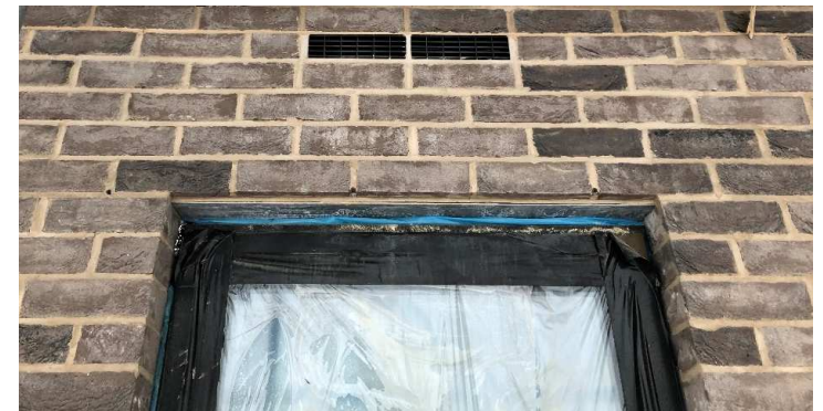
Modular Vent Brick installed over typical window (protection yet to be removed)
