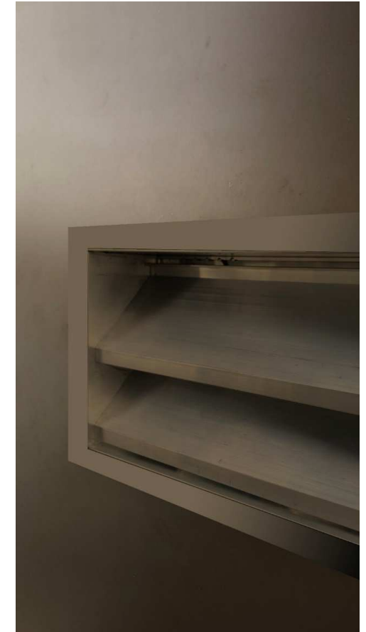
Adjusted photo to illustrate correct louvre finish with 20mm flange
