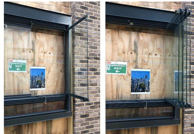
Full Sample & Opening Method of Winter Garden System ref. Window 1000 Light (incorrect finish)
