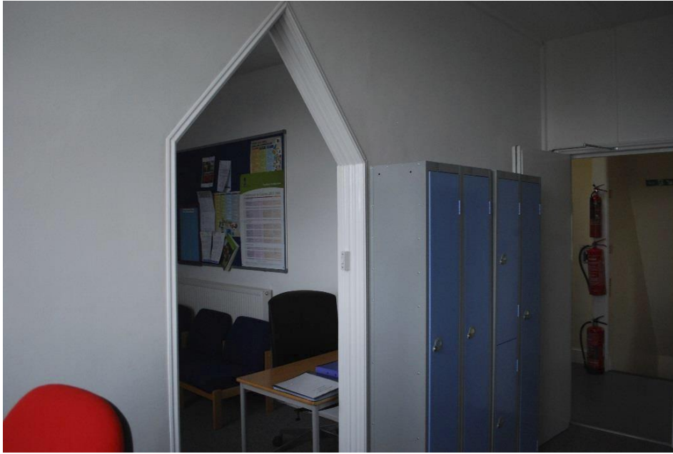
'Modern' partitions and openings at top floor level.
