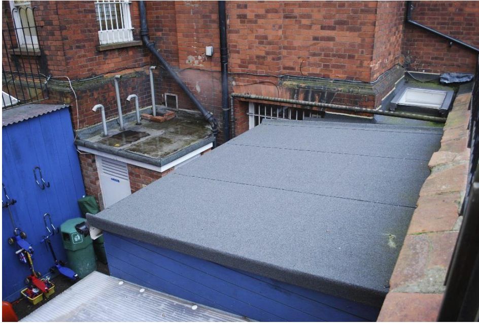
Structures in the front light-well.
